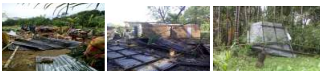
Katigorah Revenue Circle Storm damage houses.
