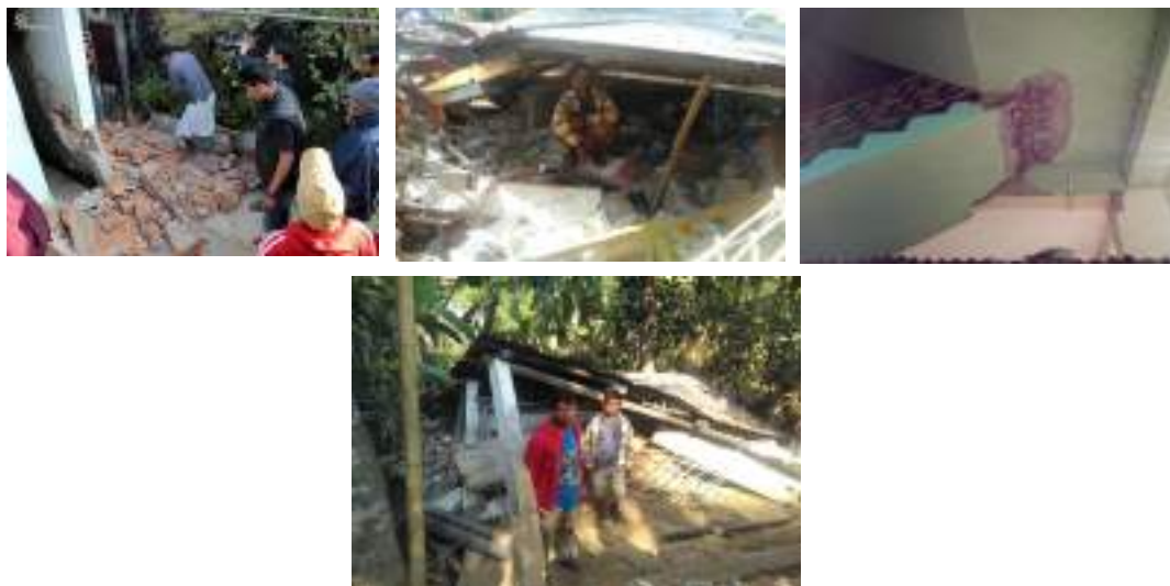
Different places of Cachar District house, flats damaged during Earthquake.
